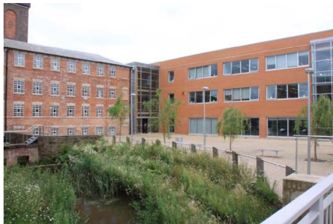
Part of the Old Mill and Part of the New School Building with the River Dove in the foreground which Powers an Archimedes Screw in the Old Mill Race Providing 80% of the Electricity for the School
