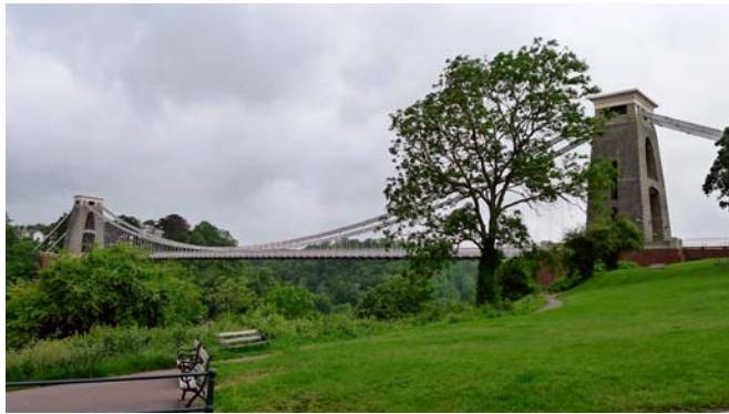
Brunel's Clifton Suspension Bridge
