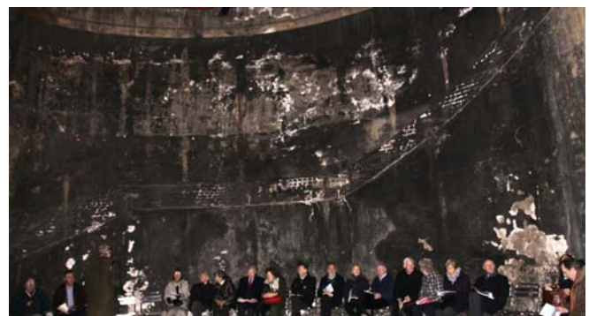
Gathered inside the Caisson which still shows evidence of the Old Staircase
