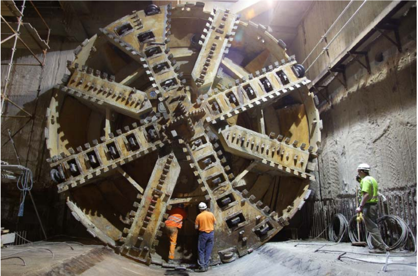
Tunnel Boring Machine
