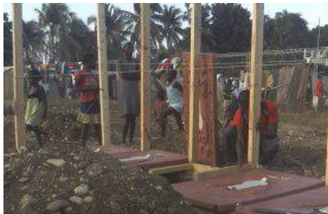
Latrine Construction in an IDP camp in Leogane
