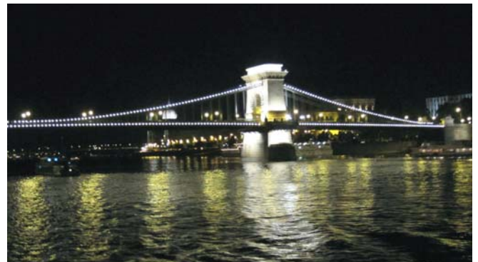
Széchenyi Chain Bridge designed by William Clark and built by Adam Clark
