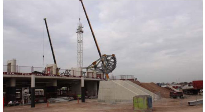
The Steelwork of the Velodrome just started
