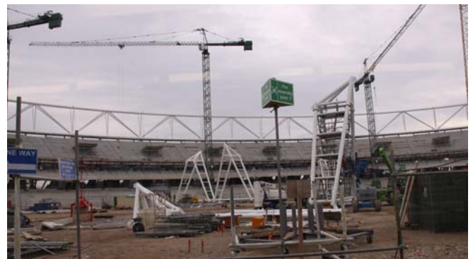
Inside the Olympic Stadium with the lighting pods being built
