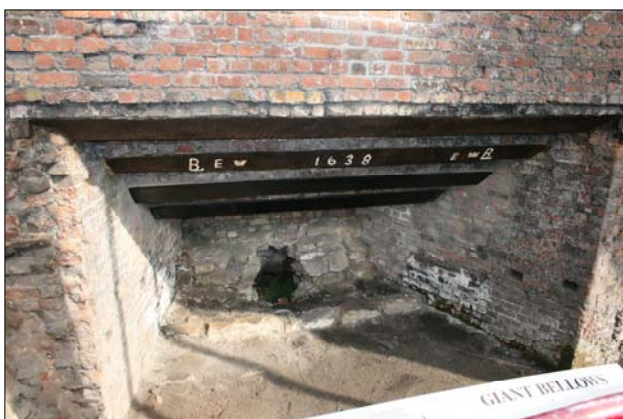
The Bellows hole at Abraham Darby’s Blast Furnace
