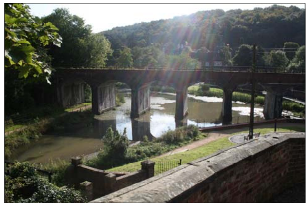
View from the Darby Houses up wind of the Furnace
