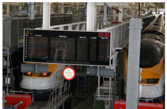
Eurostar trains in the depot for service with the information board giving the names of the train sets, the servicing regime and target completion times.
